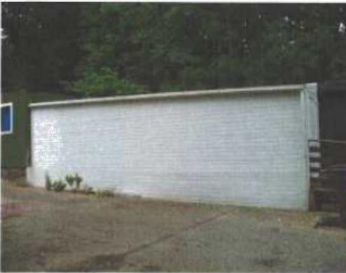
Port Cabins South-East Elevation
