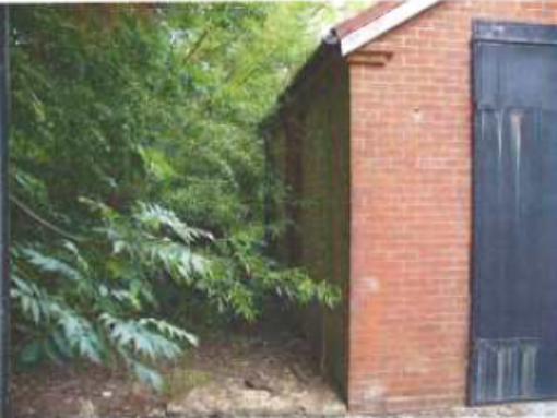
Garage North-West Elevation
