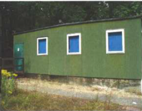
Port Cabins South-East Elevation
